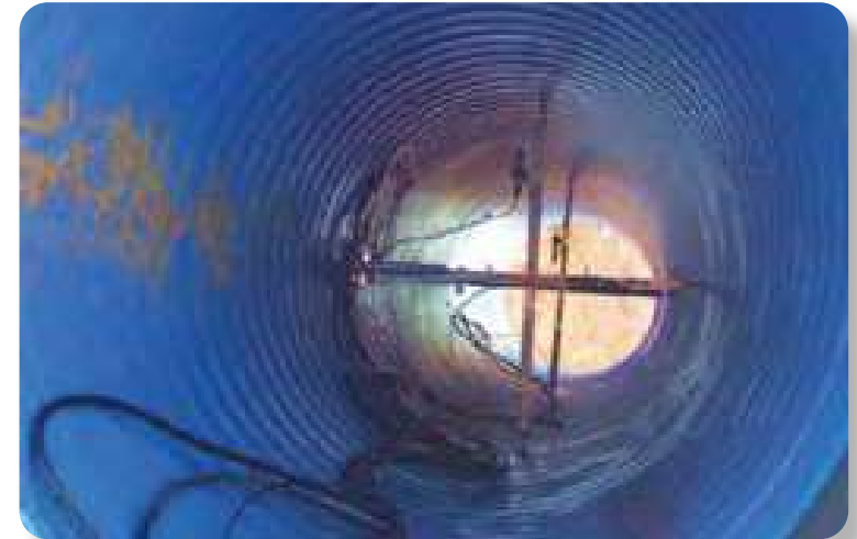
Sensors for measuring vertical and horizontal deformation
